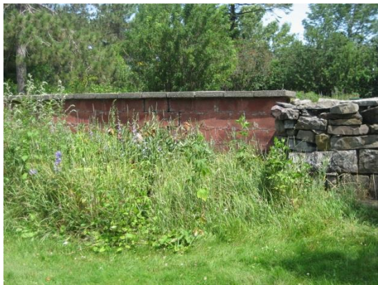
Section of Garden's Curved Wall – Before
