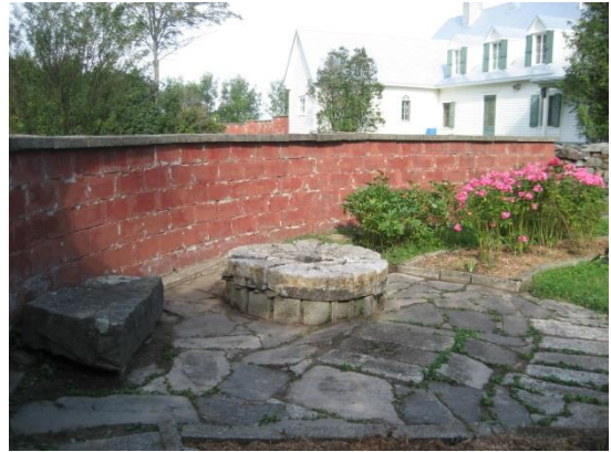
Millstone Patio - After
