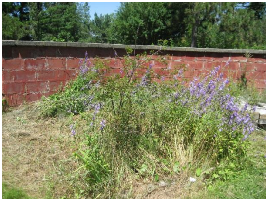
Section of Garden's Curved Wall – Before
