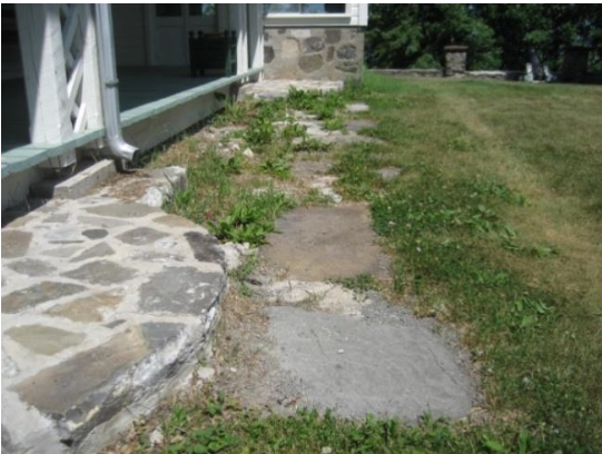
Stone Walkway at Manoir's Front Door Before
