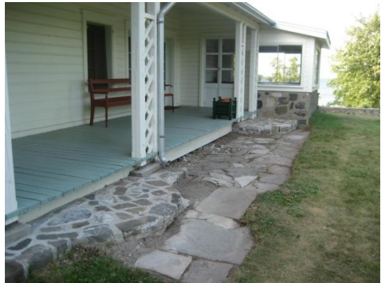
Stone Walkway at Manoir's Front Door After
